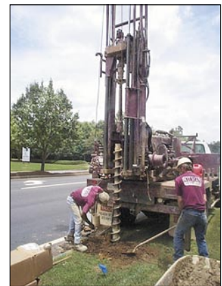
Drillers install a new regolith monitoring well. Photo by Phillip N. Albertson, USGS.
